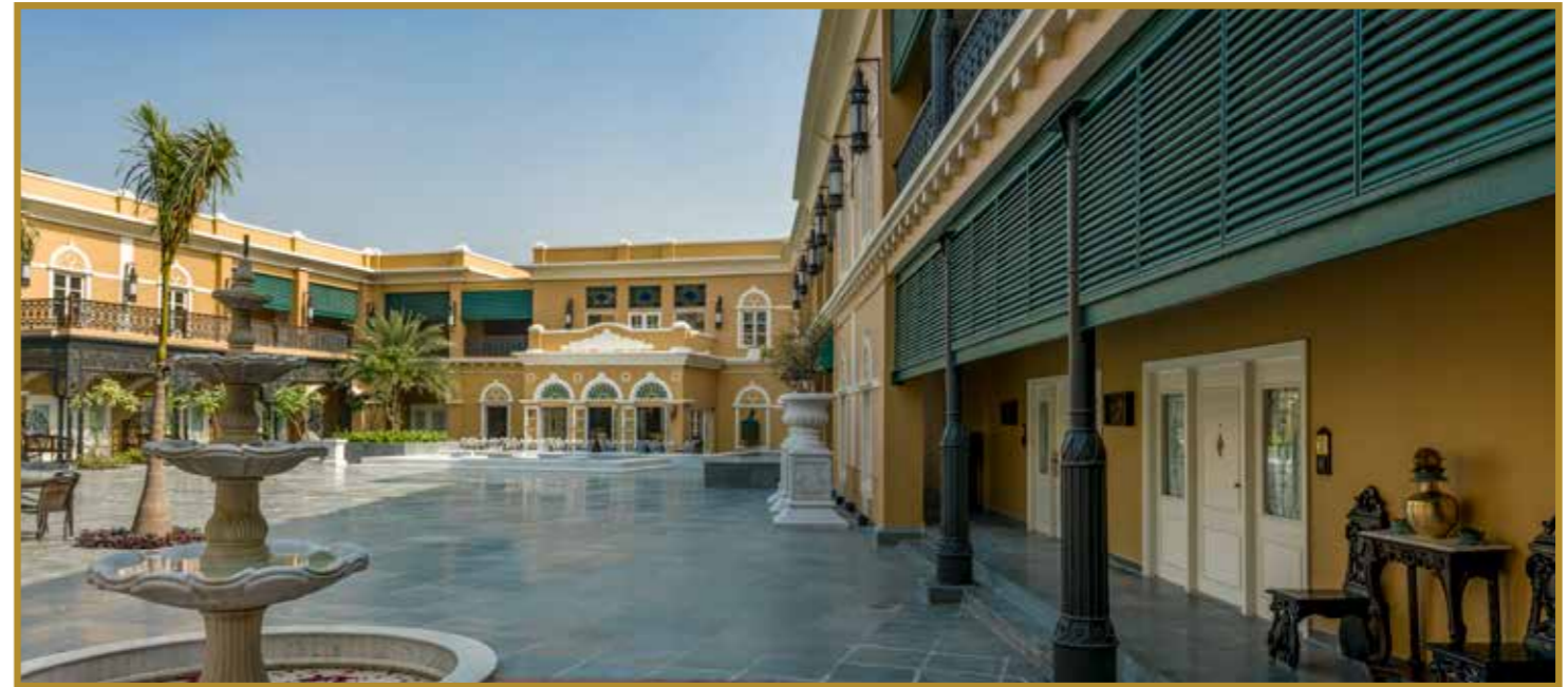
RaajKutir's courtyard view reflecting a bygone era of zamindari mansions in Kolkata
